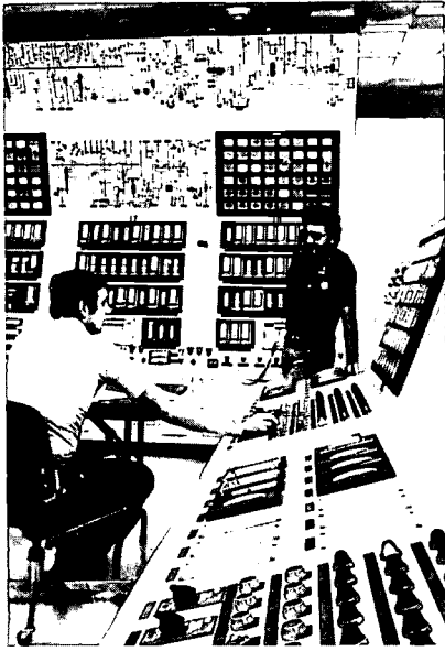
The control room is the "nerve center" of a nuclear power plant.
